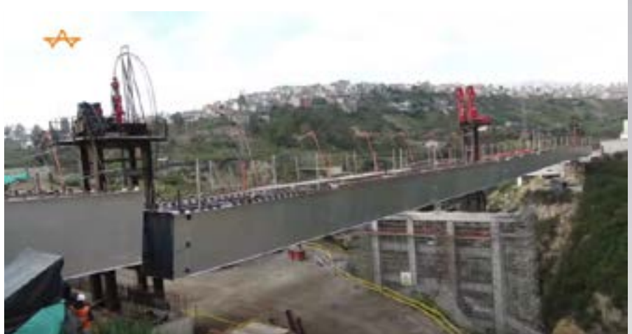
Figure 2. Bridge hanging from strand jacks during lowering operations
