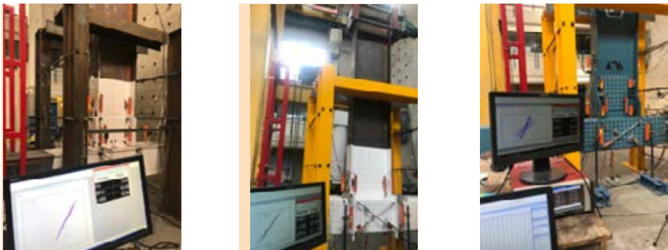
Figure 2. Specimens with wide flange beam-to-HSS column connections
